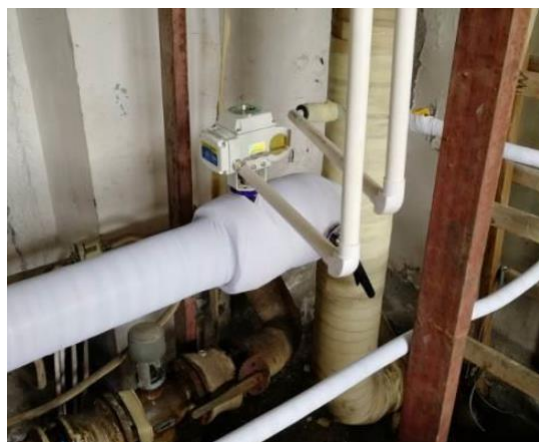
3#TES-Hybrid 動態儲冷系統配套電動閥
